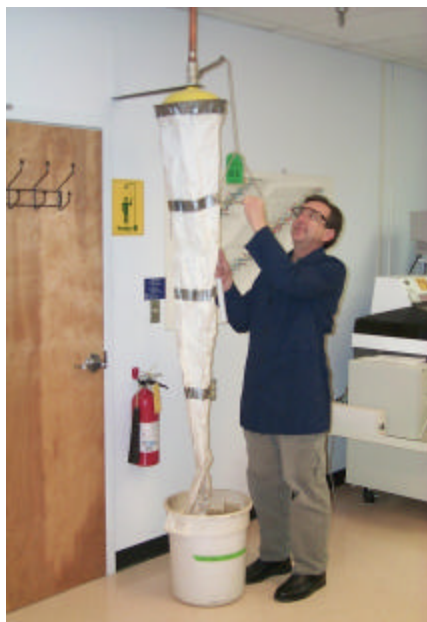
Wes Kolar, environmental safety specialist, performs yearly testing on a safety shower to ensure it is operating correctly.
