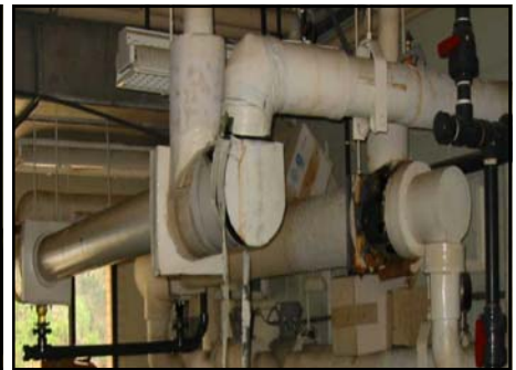
The left picture above is before the renovation in the balcony area of the marine lab. Clutter and dirty conditions are visible. Right, above is asbestos-covered pipes which are in dire need of repair, for safety as well as appearance.
